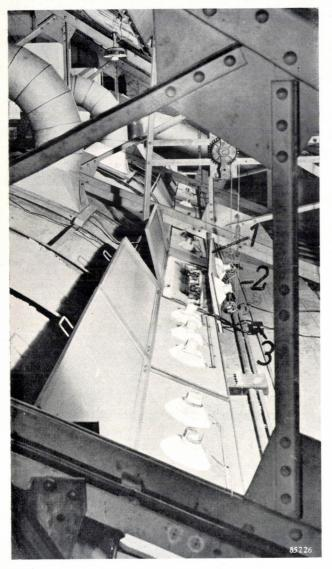
Fig. 9. The loudspeakers of the stereo reverberation installation in the Philips Theatre are mounted in groups of two or three in the panels which cover the lighting cornice (L in fig. 6). At l one of the panels has been lifted up. 2 is the (sixcore) cable, 3 a junction box.
