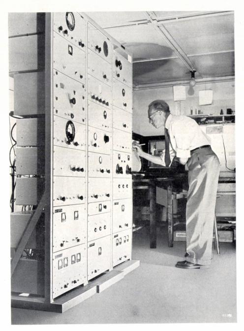
Fig. 8. The radio receiver as installed at Kootwijk.
