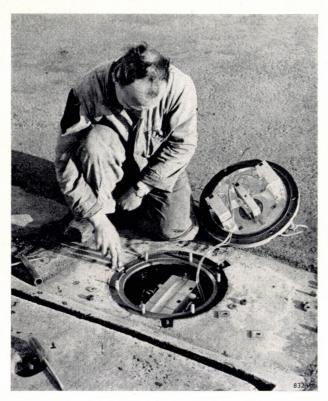
Fig. 13. Three transformers of the simplest type mounted in a flush runway light (as shown in fig. 21 of the article referred to in note 1)). The cover, only the bottom of which is seen in the photograph, contains one omni-directional top light and two beam lights (one for each landing direction).
